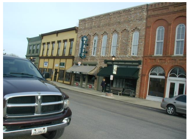
The Palms Grill Café Restoration Work Completed 2009
