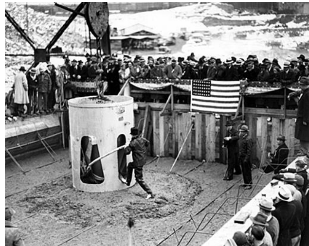
Picture 1: Construction underway at Grand Coulee Dam Source: U.S. Fish and Wildlife Service
