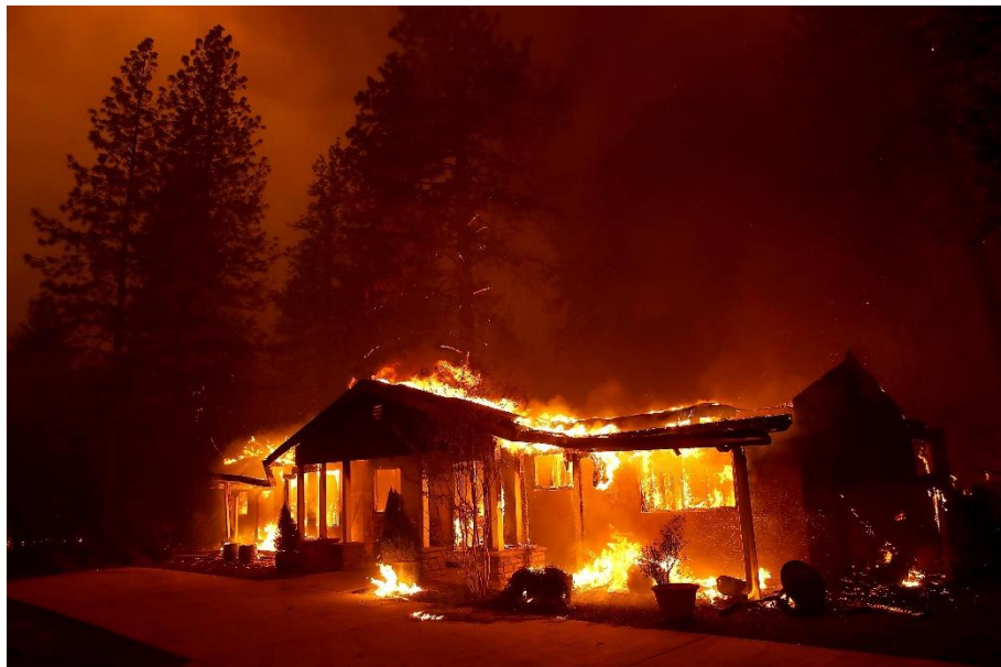
Home destroyed by Camp Fire in Paradise, California.
