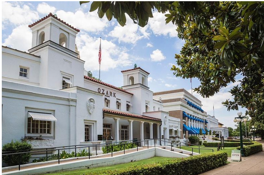
Bathhouse Row in Hot Springs National Park. Source: Arkansas Democrat Gazette, 2021.
