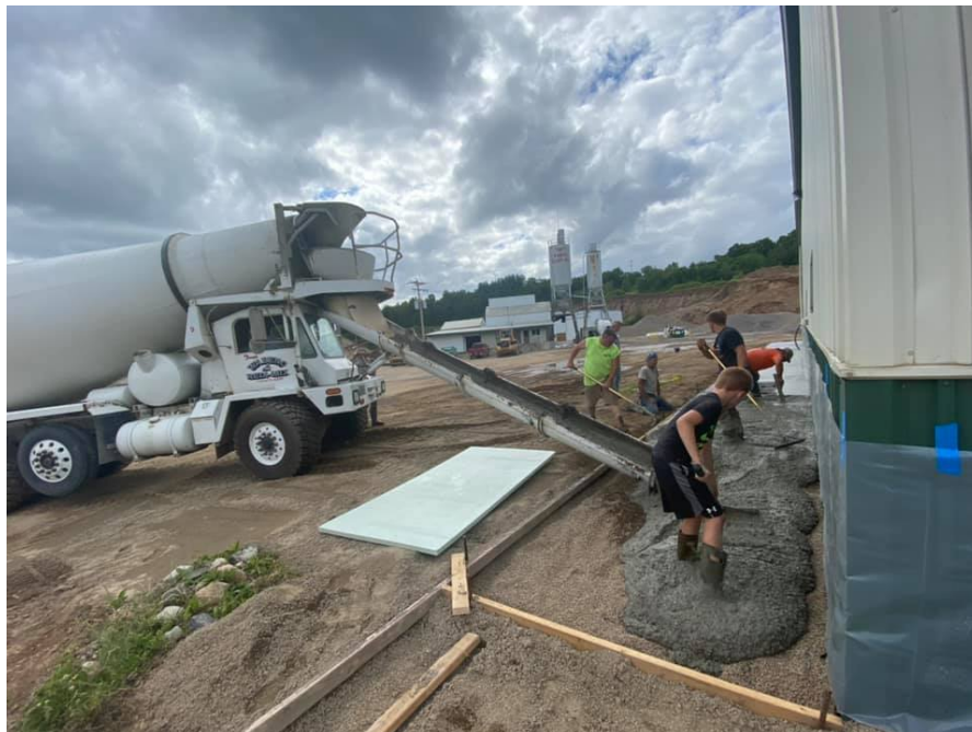
The concrete being poured in this photo is derived from aggregates. Source: Tony’s Wabeno Redi-Mix, LLC, 2020.
