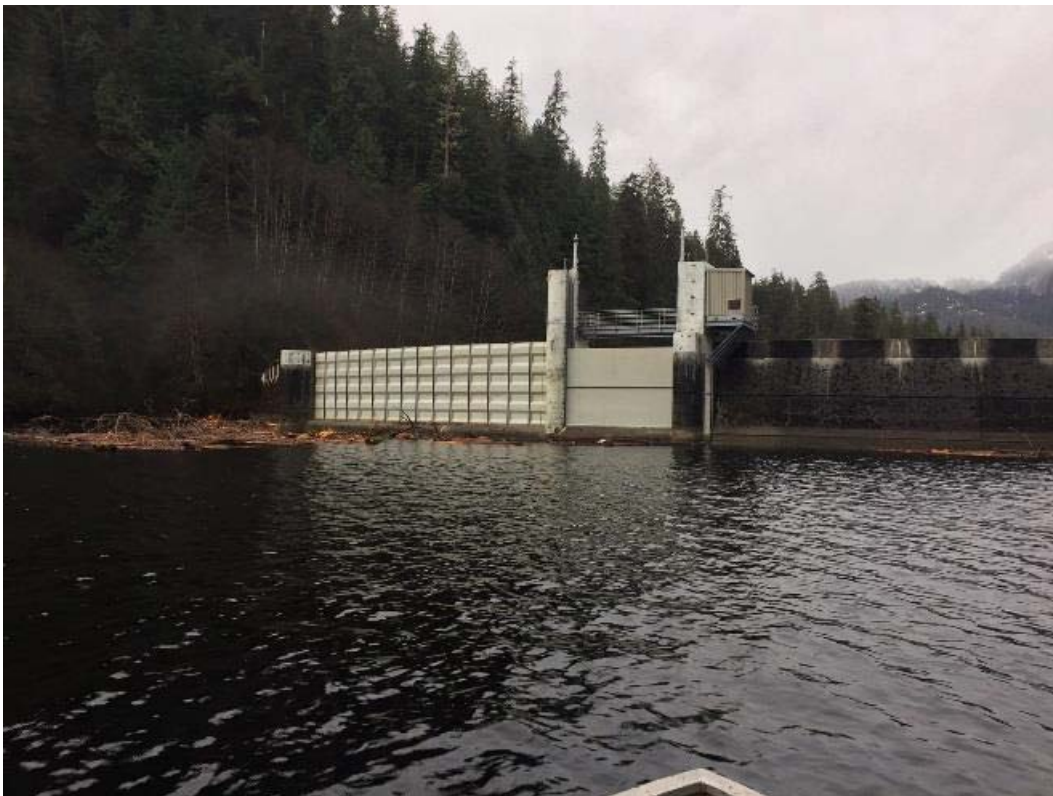
Spillway Construction Complete – 15 Foot Reservoir Elevation Increase
