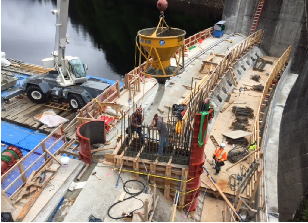
Middle Pier Concrete Placement
