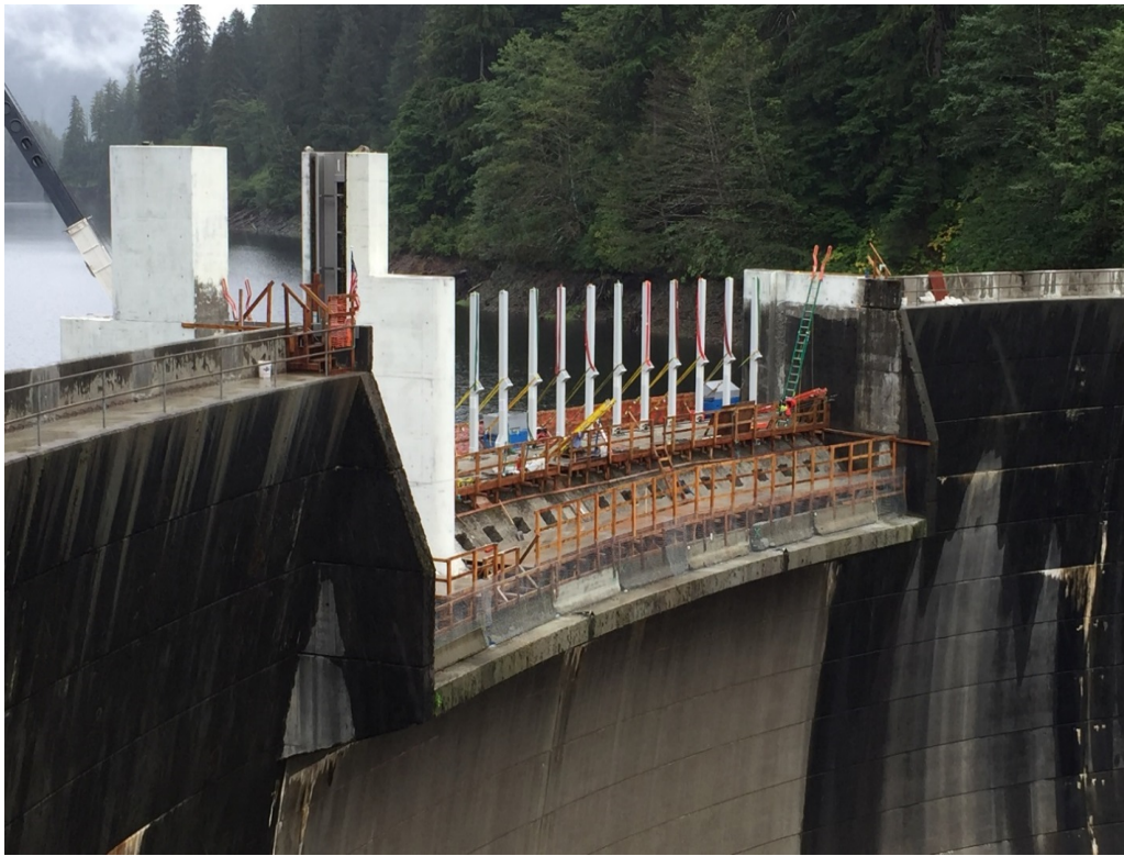
Gate Piers Complete – Flashboard Columns Erected
