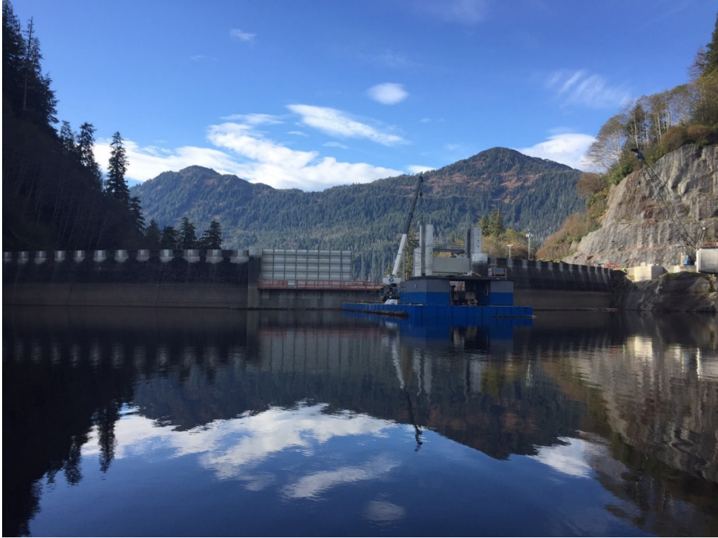
Crane on Barge – Placing Flashboard Panels and Vertical Gate
