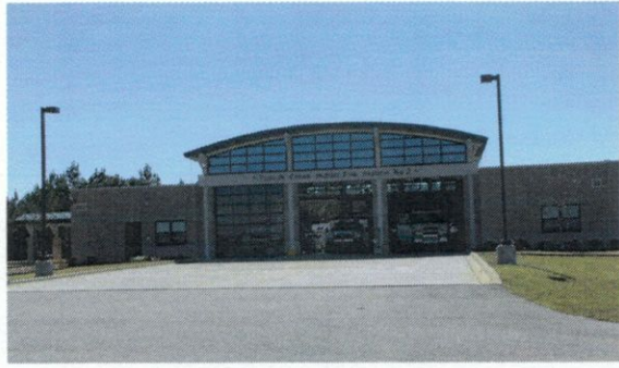
Poarch Creek Fire Station Located on Poarch Creek Fee Land
