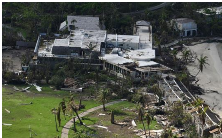
Caneel Bay damage post-hurricanes – Photo by the Federal Emergency Management Agency
