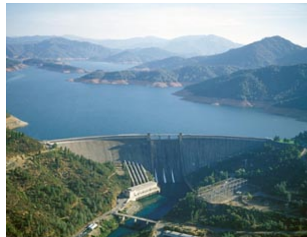
Figure 4 Picture of Shasta Dam, a vital part of the Central Valley Project. | Source: National Park Service
