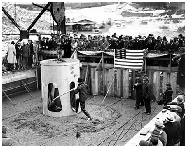
Picture 1: December 6, 1935. Washington Governor Clarence C. Martin placing official first concrete pour at Grand Coulee Dam. | Source: U.S. Bureau of Reclamation
