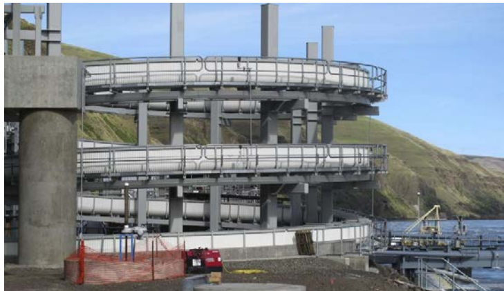
Picture 2: Picture shows fish ladder at Lower Granite Dam. [Source: Nicholas K. Geranios/Associated Press File
