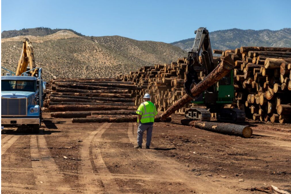
The Washoe Tribe of Nevada & California is working with private partners and the FS to build a sawmill to help process salvage and excess fuels. Source: Tahoe Fund, 2022.
