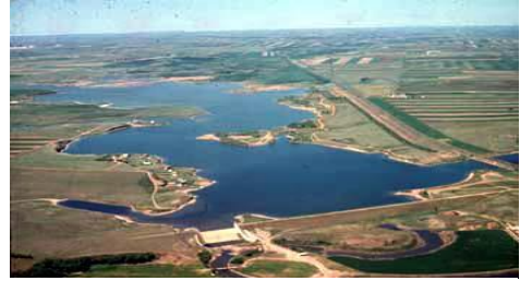
Dickinson Dam and Reservoir. Photograph provided by the Bureau of Reclamation
