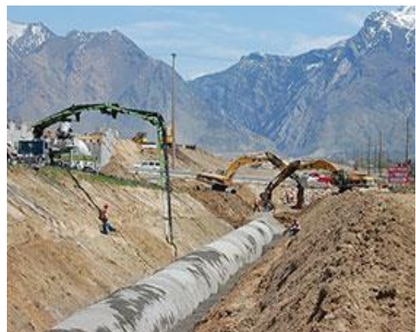
Picture 1: Piping of the Provo Reservoir Canal in Utah, Source: Bureau of Reclamation, Upper Colorado Region
