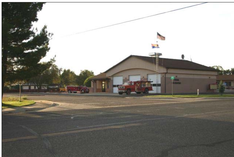
Figure 6. Fire Station in Fredonia, Arizona
