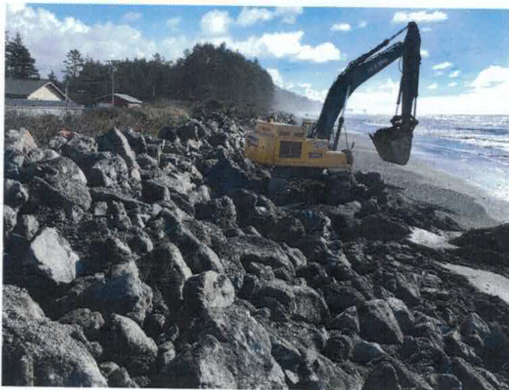
Building the temporary break wall
