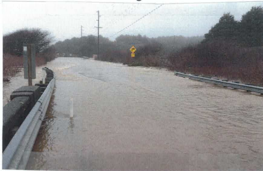
Quinault River washing over the only access road during a storm
