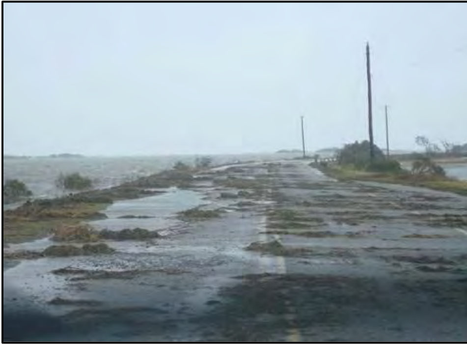
Figure 4. Post-Storm Beach Road, which provides access to the beach parking lots, November 2009.
