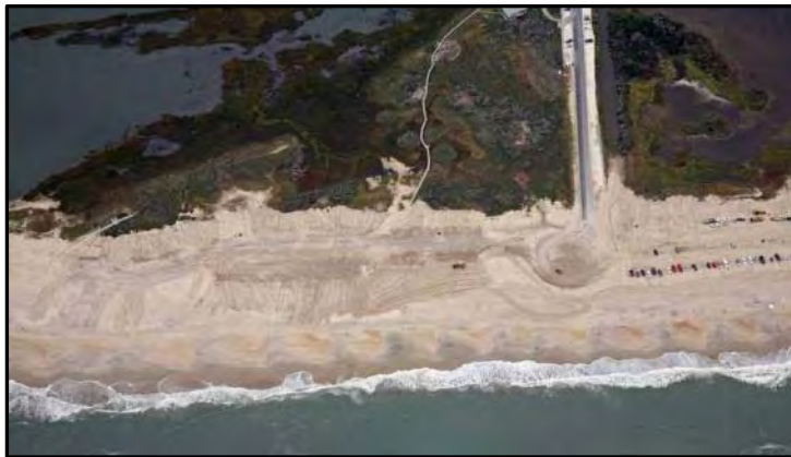
Figure 5. Damage and Clean-up of Parking Areas 2-4.
