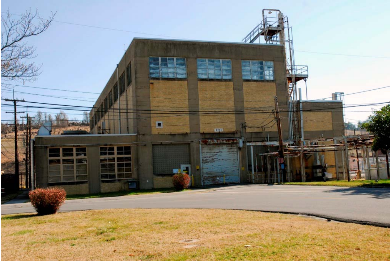
Building 9731, Y-12's Pilot Plant
