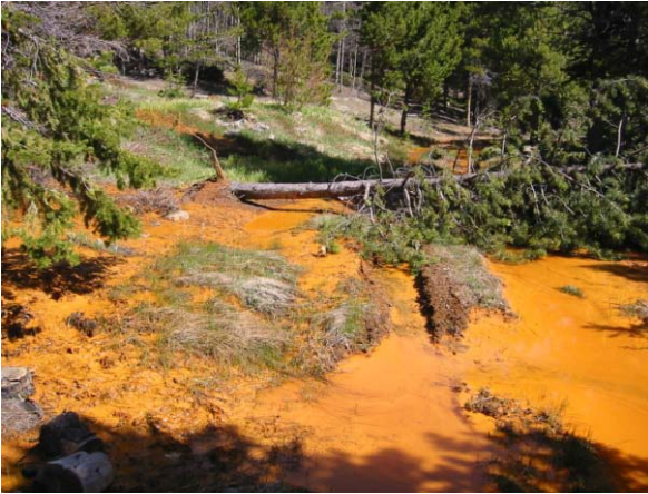
Figure 2 - Perigo Mine, Gilpin Co, CO Adit
