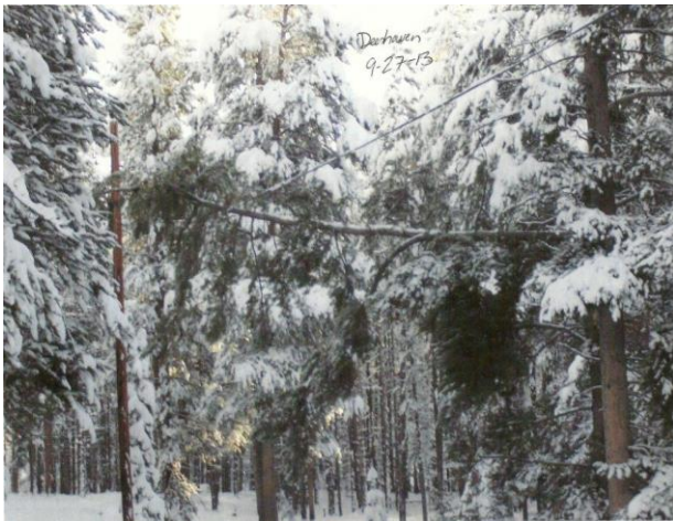
Photo 2: Tree Leaning on Distribution Line in the Big Horn National Forest. Source: Big Horn REA
