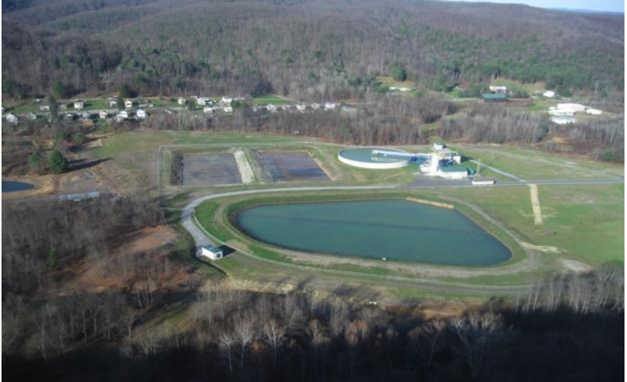
Aerial view of the Hollywood AMD Treatment Plant
