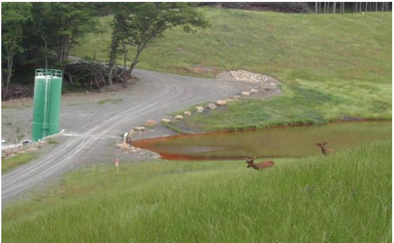
Lime Doser Treating Abandoned Deep Mine Discharge in the Bennett Branch Watershed
